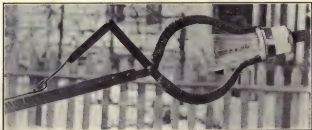
FIG. 1.—Construction of device for replacing street lamps.
